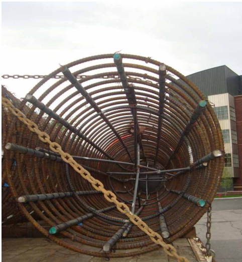
Figure 1. X-Brace Configuration
