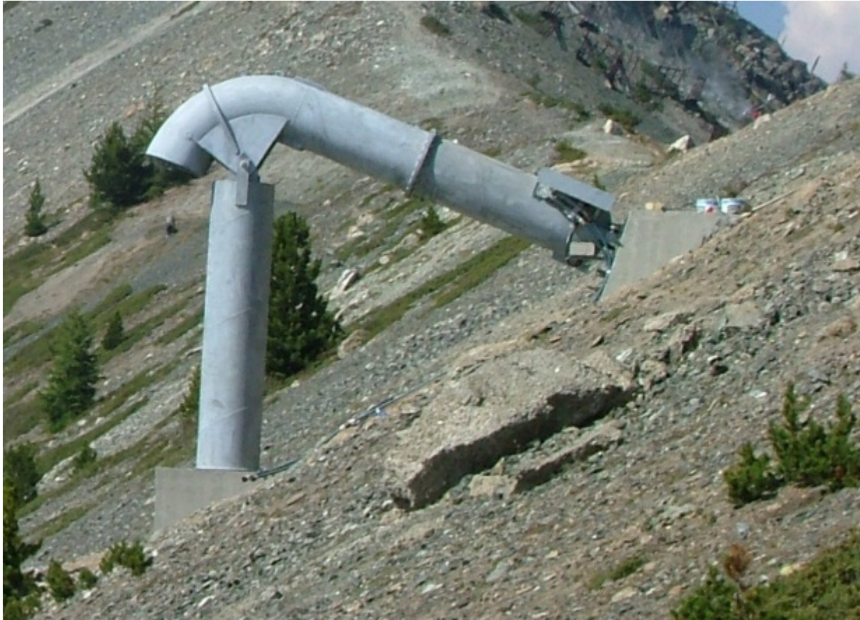
Figure 1. A Gazex system in Colorado. Cylinders of oxygen and propane are stored in the cement bunker at the base of the exhaust piping. The gases are ignited and the resulting shockwave is directed over the top of the snow in avalanche-prone areas.
