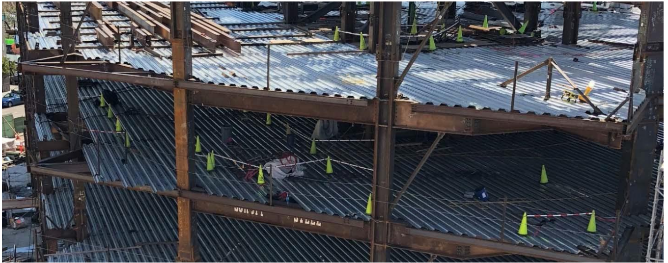
Picture 1: Bar and cone barrier system in use
