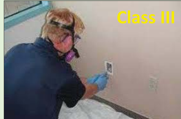
Repair and Maintenance
