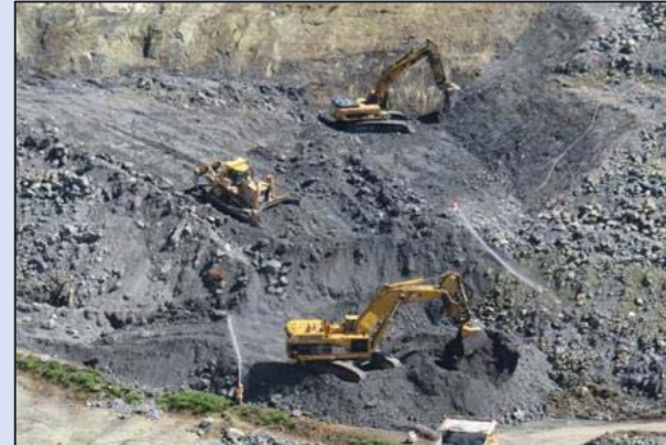
Excavation of Loose Material
