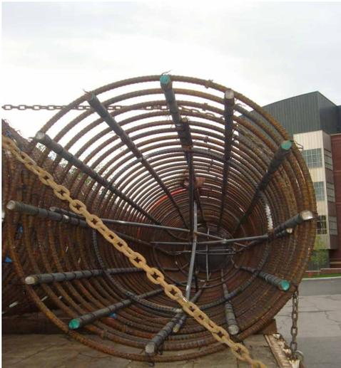
Figure 1. X-Brace Configuration
