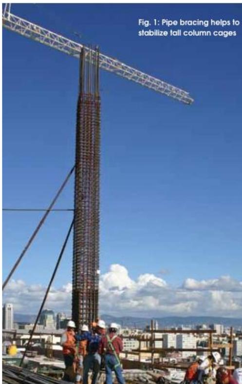
Fig. 1: Pipe bracing helps to stabilize tall column cages
