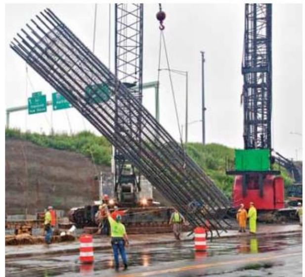
Fig. 7: A well-braced drilled shaft cage is picked with minimal distortion (photo courtesy of Dimension Fabricators, Inc.)
