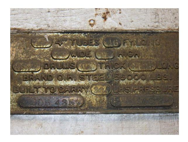
This boiler displayed a second nameplate to list the specifications: (252) 4'' tubes; 16 ft. long; (3) 12' drums,  $\frac{1}{2}''$  thick; Built 1903. The boiler produces steam used for drying paper at various stages in the paper-making process.
