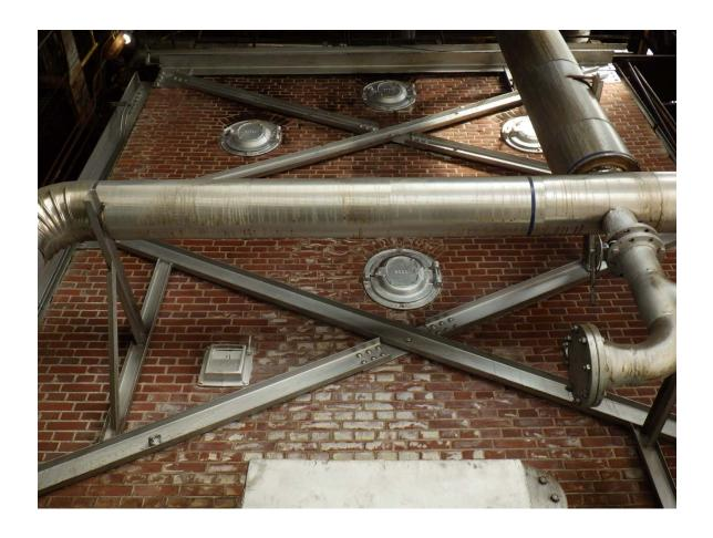
Boiler #5, along with boiler #2 are the workhorses for PABCO. This Stirling boiler is duel-fired (oil and gas) and once utilized a superheater, which has since been removed.
