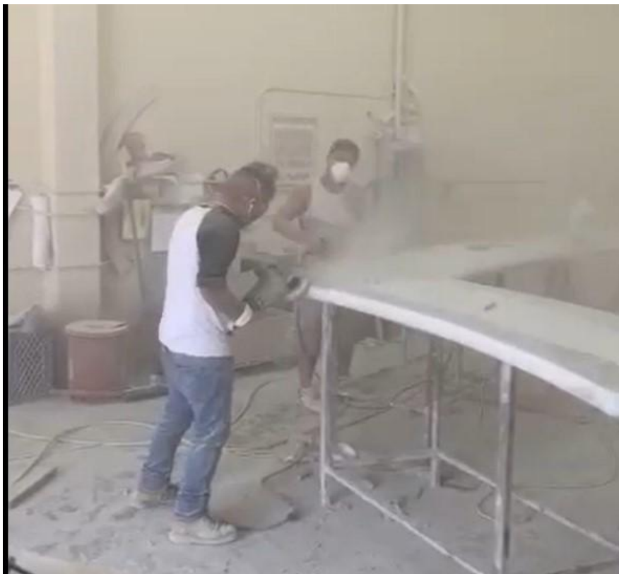
Plate 1. A worker performs grinding or polishing on a countertop edge. A dust plume is visible at the tool. No water suppression and no local exhaust capture are in use at the work position. The operator has no respiratory protection. Dust has accumulated on the floor, the work surfaces and the walls.
