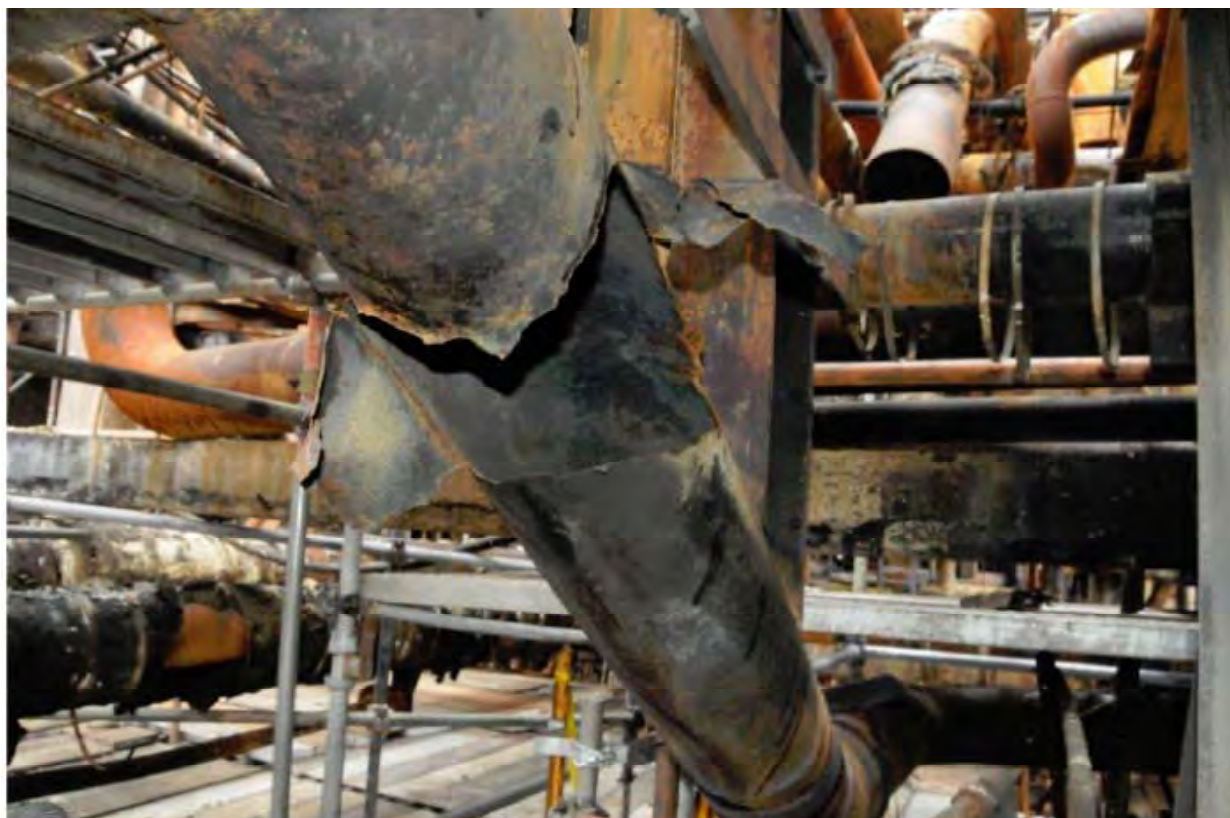
Figure 5. Photo of rupture on 4-sidecut 52-inch component.
