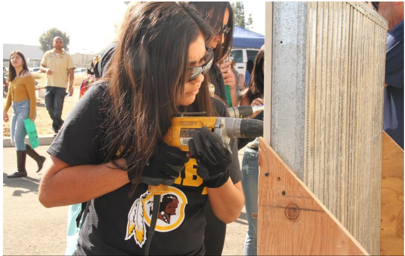
A high school student drills drywall to metal studs at the Student Apprentice workshop during National Apprenticeship Week.
