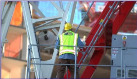
Inspecting unusual places
