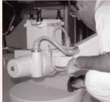
Clean and decontaminate the worksite.
