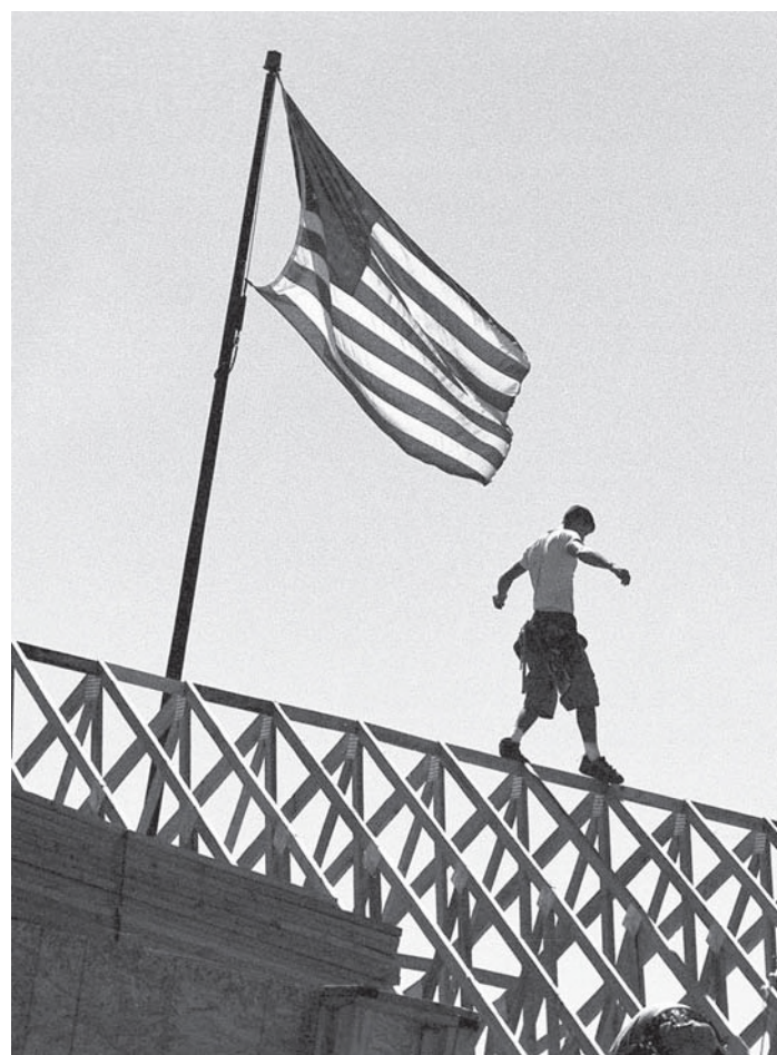
DLSE and Cal/OSHA investigators conduct enforcement sweeps in residential construction projects to combat widespread labor law violations. This residential construction worker should be wearing fall protection to prevent a potentially fatal accident.
