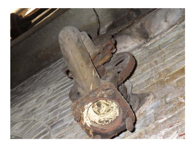
A view of an early sootblower design that has been disconnected for many years due to environmental regulations. Today, the boiler operator cleans the boiler cavity "by hand" using a portable pressure washer when maintenance is due.
