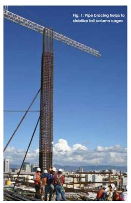
For larger column cages, greater than about 36 in. (910 mm) OD, X-bracing is added to supplement the inner hoops. The brace locations are usually provided by two reinforcing bars with a Type 19 bend pattern.<sup>3</sup> They are then placed perpendicular to one another in a three-dimensional fashion, located in the column cage interior. The bar size is usually two sizes smaller than the longitudinal bars, but this can vary by shop practice and experience.
