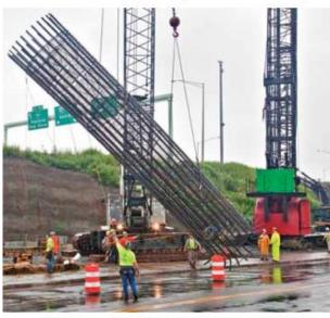
Fig. 7: A well-braced drilled shaft cage is picked with minimal distortion (photo courtesy of Dimension Fabricators, Inc.)
