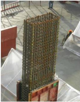
Fig. 2: A column cage with many large vertical bars and crosstles can be stable enough to eliminate the need for
