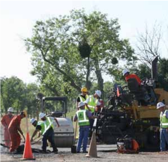
Local 3 apprentices pave the entrance to the new training site in April.
