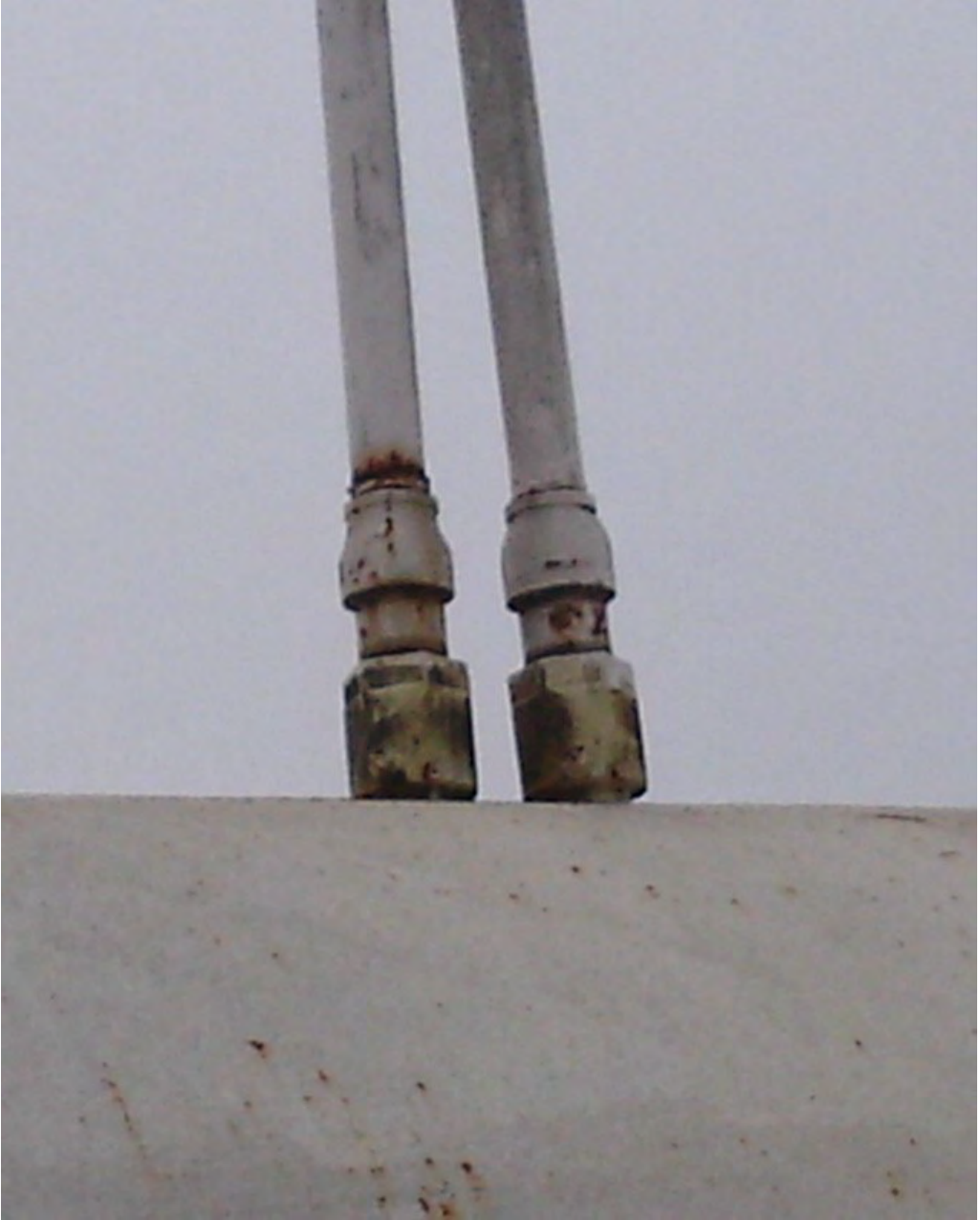
In both pictures the outlet of the relief valves is restricted.
