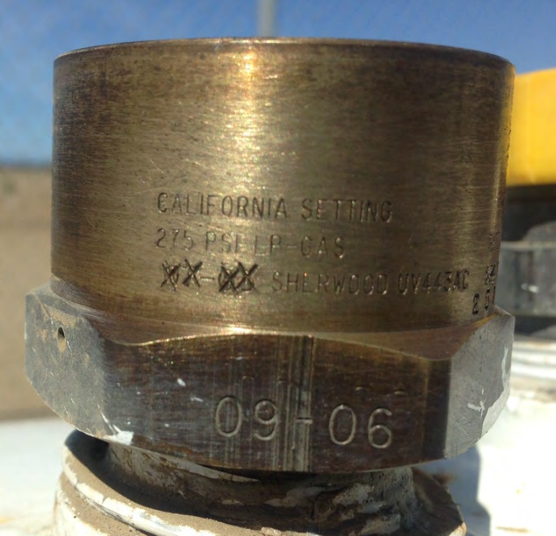
Sherwood – Dual Stamped LP-Gas safety relief valve. When inspecting tanks with these valves, record the set point as 250 psi.
