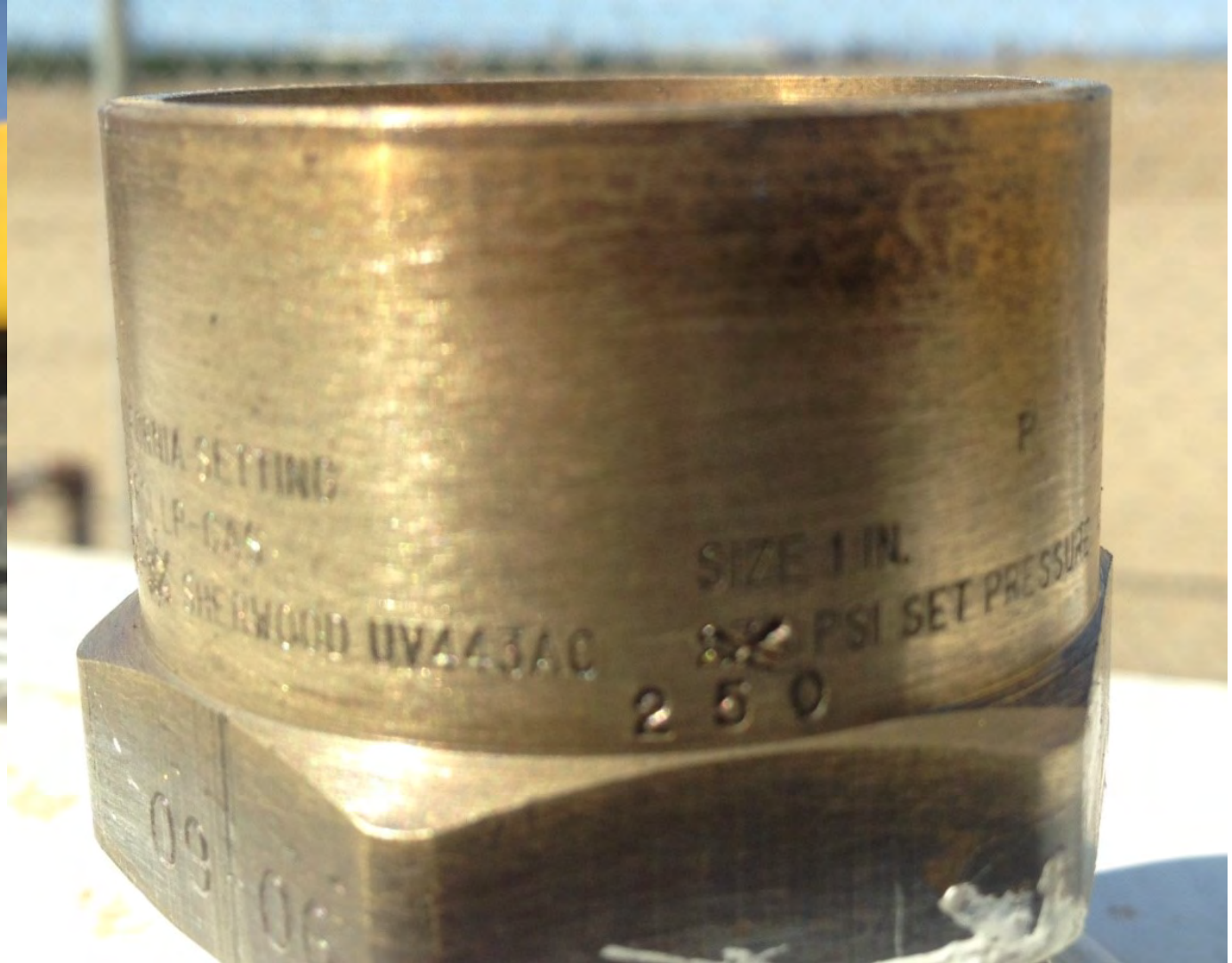
Sherwood – Dual Stamped LP-Gas safety relief valve. When inspecting tanks with these valves, record the set point as 250 psi.
