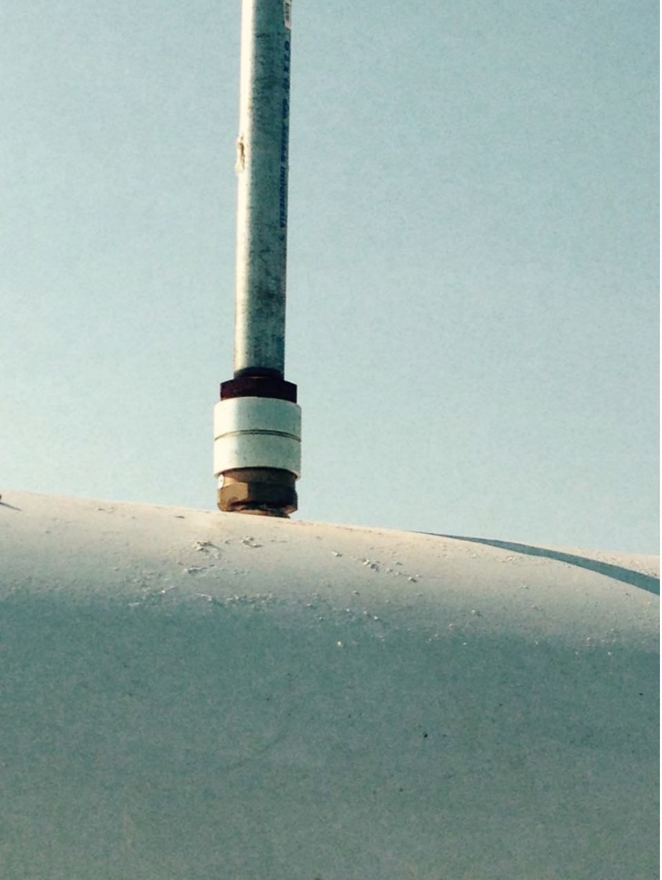
In both pictures the outlet of the relief valves is restricted.
