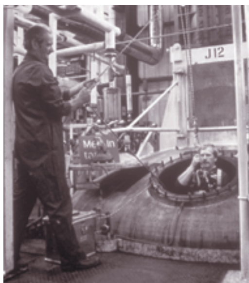
Entrance into confined space with assistance of an attendant
