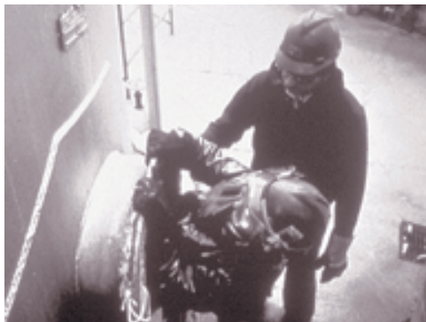
A worker crosses the plane of entry into a confined space.
