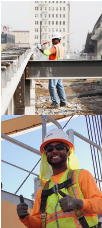
Top photo: Demolition work on the Tuolumne Street Bridge in Fresno. Bottom photo: Apprentice Arlan Harrell, who is also the subject of the cover photo, gives a positive sign at the Highway 145 worksite in Madera.
