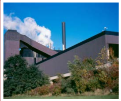
Grate-Fired Refuse Boilers
