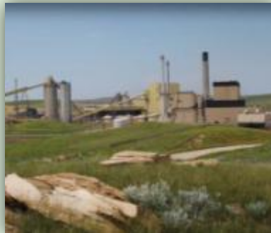
Total Environmental Solutions for Utility & Industrial
