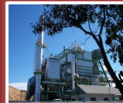
BFB Boilers and WtE
