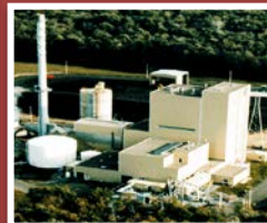
CFB Boilers and WtE
