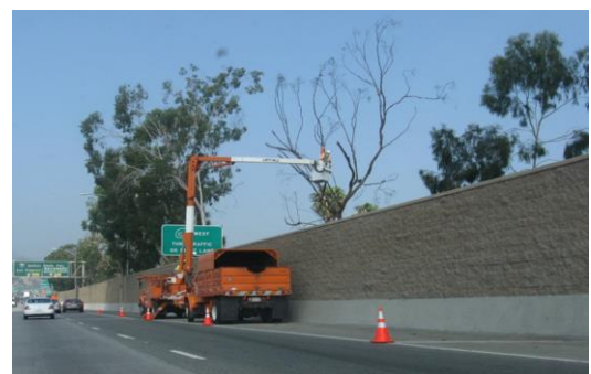
Traffic warning cones establish drop zone
