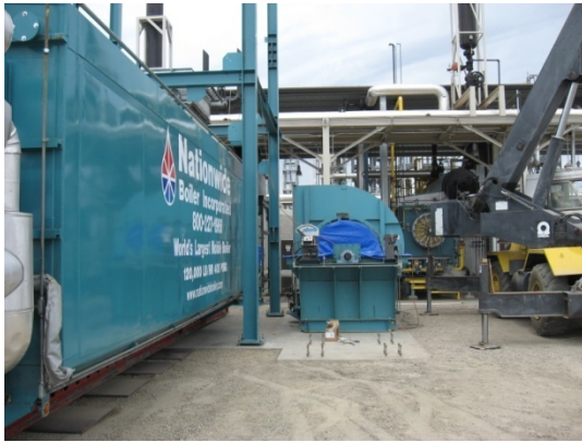
engineered fill & concrete
